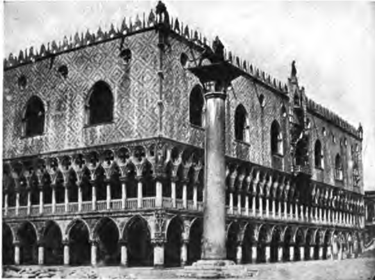
A characteristic Italian rendering of Gothic architecture, rich in the colour, detail and surface decoration later seen in Renaissance architecture (The Palace of the Doges, Venice)
